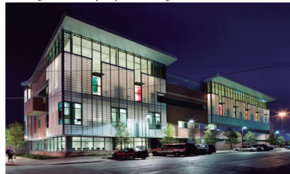
Figura 10: Fachada principal do The Bridge Homeless Assistance Center.
