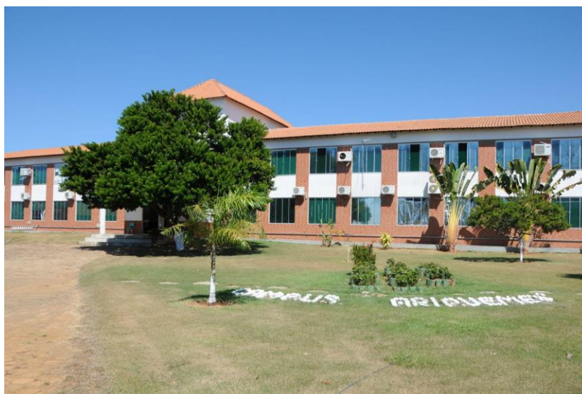
Figura 2 - Fachada IFRO Campus Ariquemes
